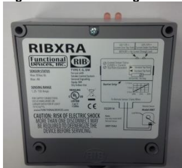
Figure 20: Flow Proving Device
